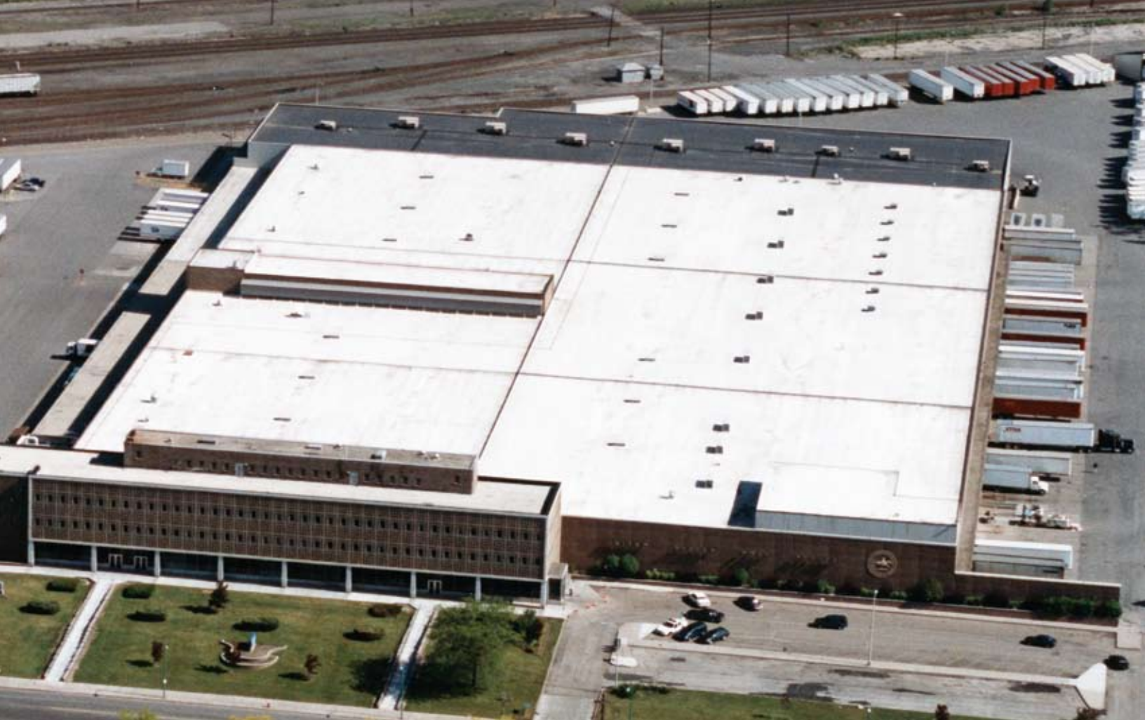
▲ United States Postal Service facility, Buffalo, NY.
