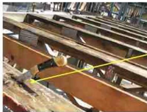
Figure 2: Decaying Timber is soft and spongy and can easily be penetrated with a knife or screwdriver
