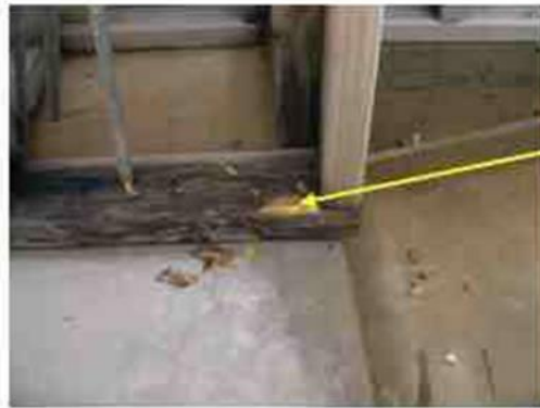
Figure 1: Although heavily discoloured with surface mould and blue stain, the pine timber is still sound as shown by scraping back the surface layer
