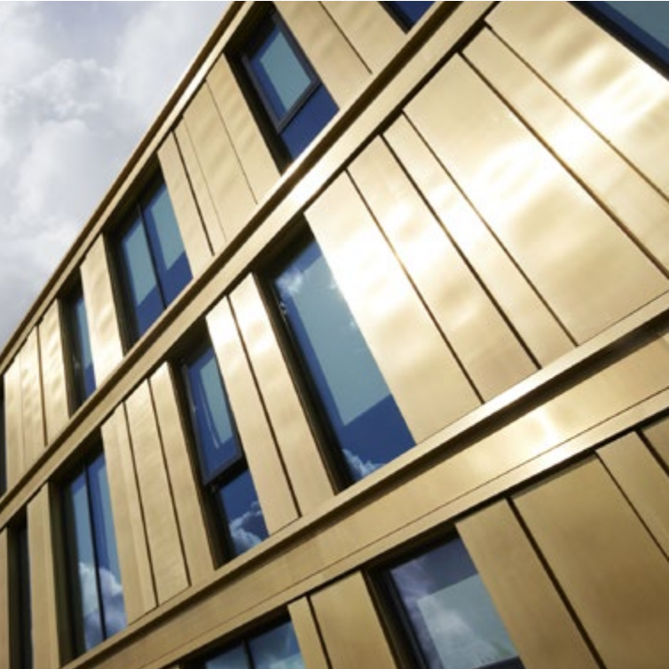
Brass Cladding Cassettes Ruuki and Vimpeli
