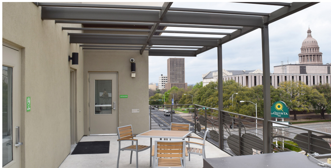
Left: Lakeline multi-family development Construction site. Right above: Transportation board located at M Station. Right: Shared balcony space at Capital Studios.
