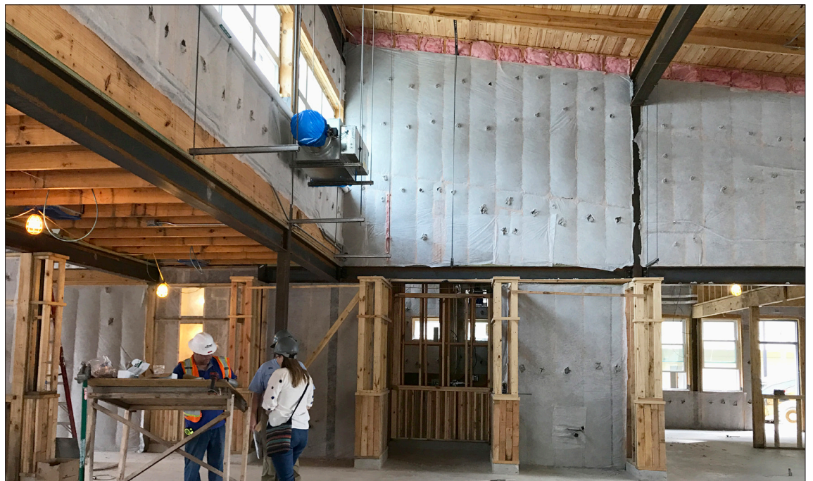
Right: Lakeline learning center construction site. © Foundation Communities Right page: M Station learning center in use.
