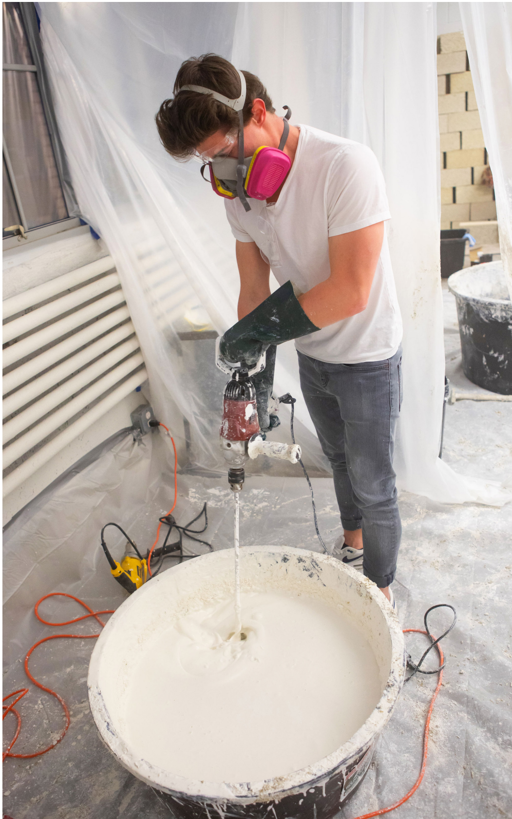
Fig 1.2 Lime and Water Mixture
