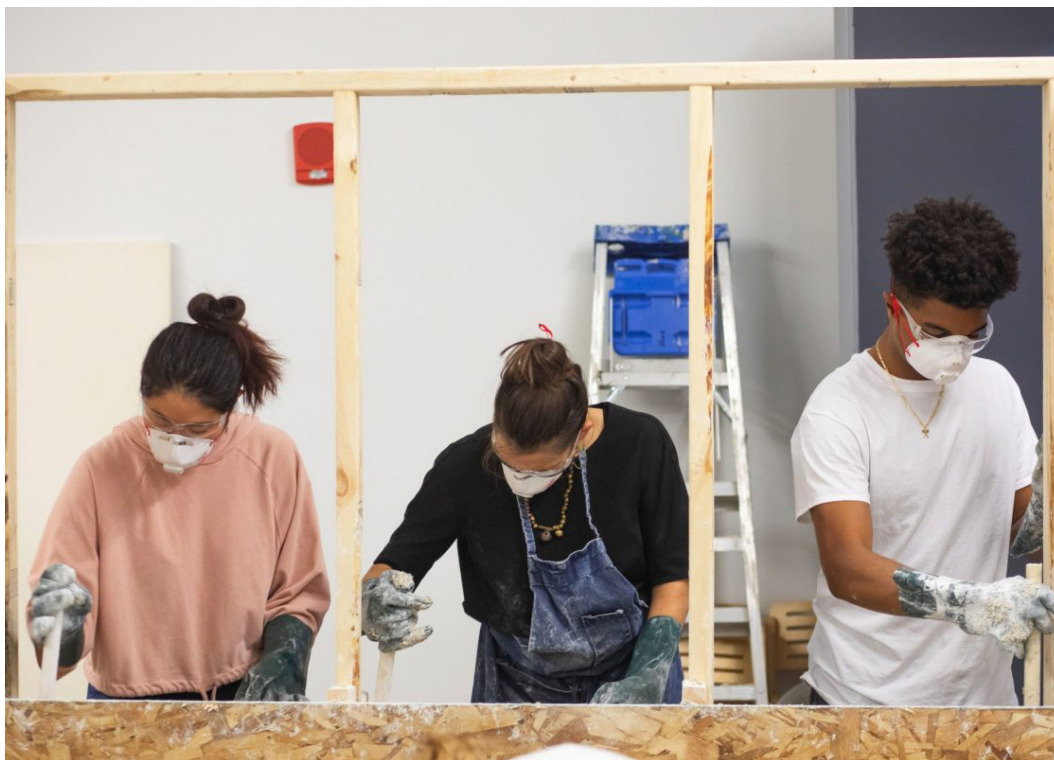
Fig 1.5 Tamping down Hemp and Lime into framework for a cast-in-place wall
