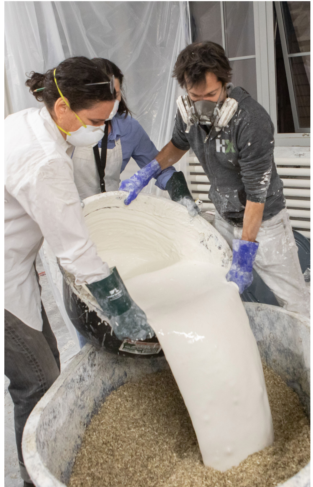
Fig 1.3 Lime and Water being mixed with Hemp
