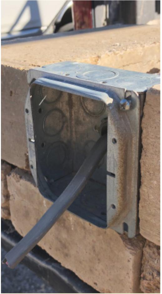
Electrical box placed in the wall during construction with conduit placed between the two wythes of blocks.
