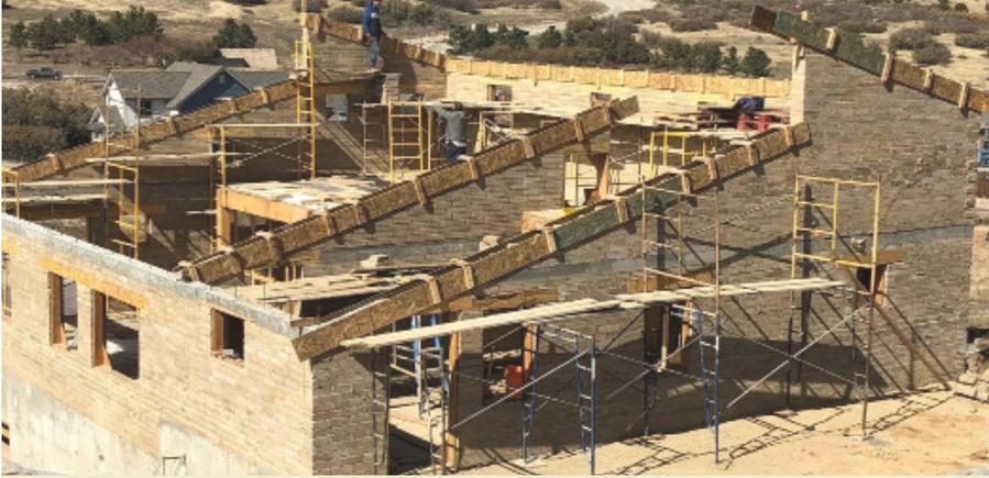
Exterior walls under construction with formwork for poured, reinforced concrete bond beam at the top of the wall and between floor levels.
