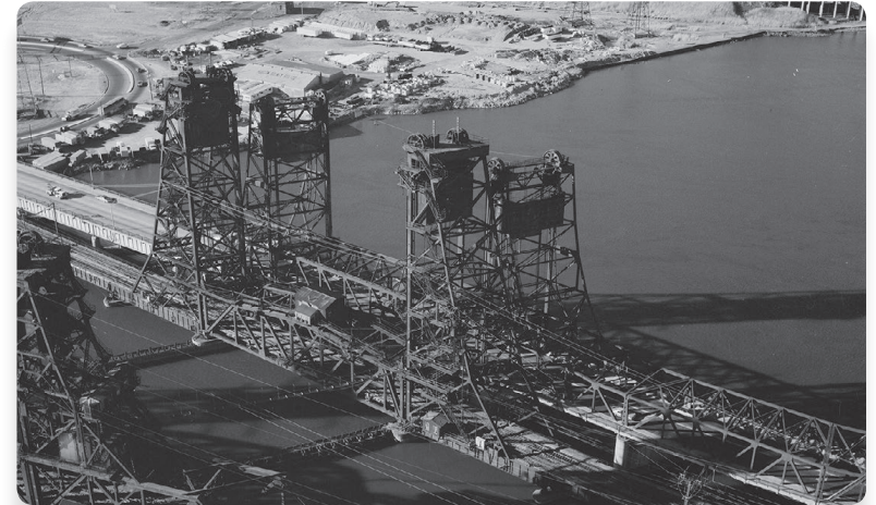
Top: Pennsylvania Railroad Harsimus Branch Bridge, as it appeared in 1928, at the center of the photo. Photo from Historic American Engineering Record: NJ-43, "Conrail Bridge, Spanning Hackensack River, Kearny, Hudson County, NJ," Courtesy of the Library of Congress.
