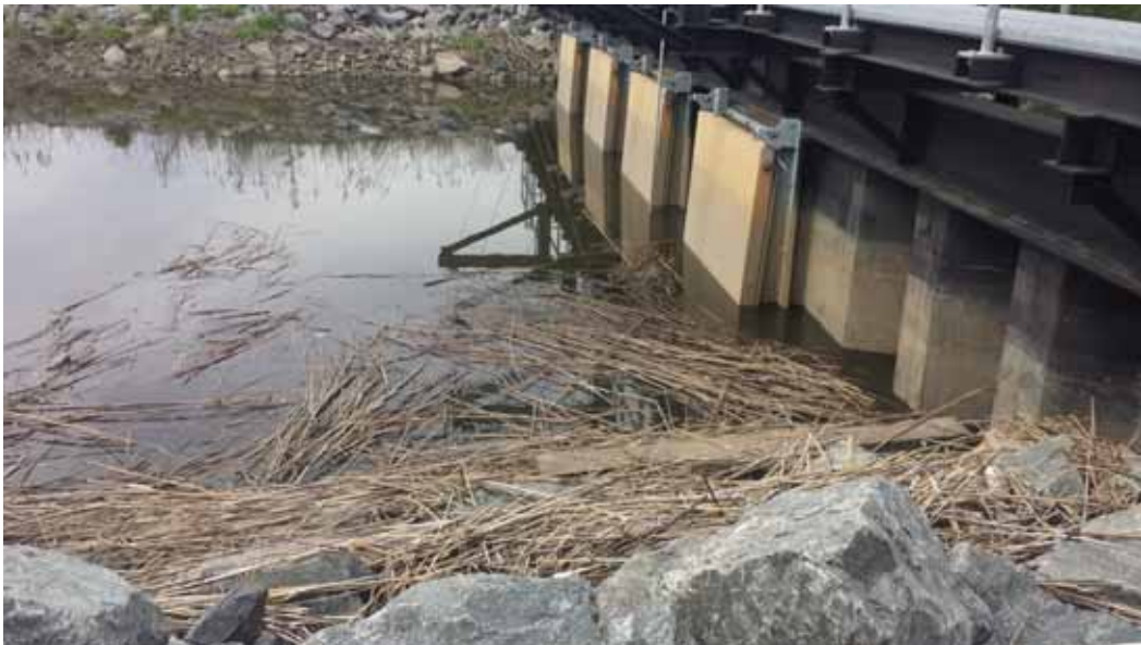
Figure 2: Side view of tide gate downstream
