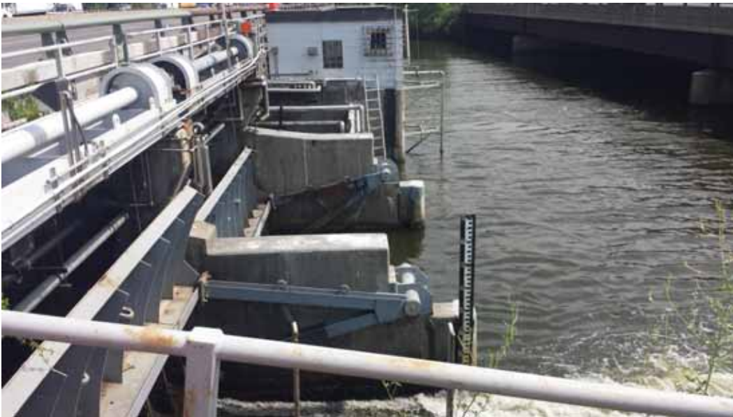
Figure 6: View of one bascule gate in operation from south of control room
