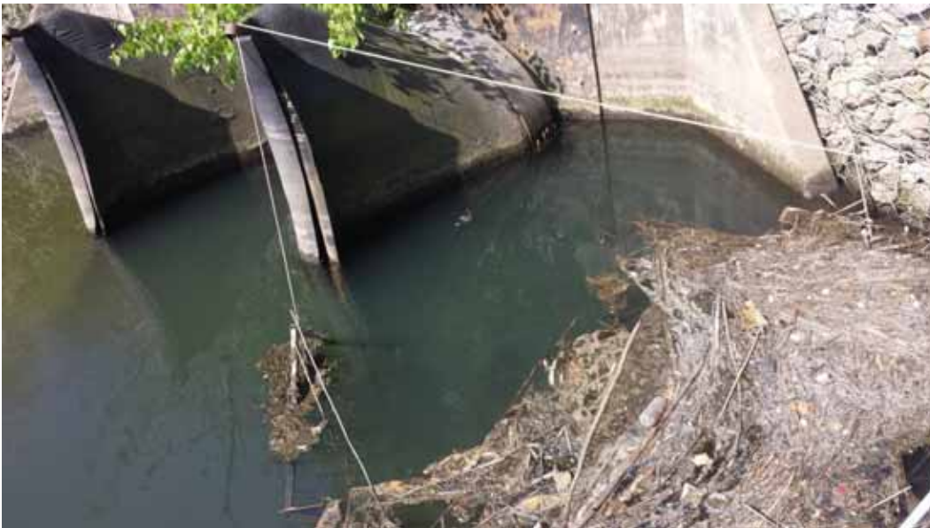
Figure 2: Upstream view of tide gate
