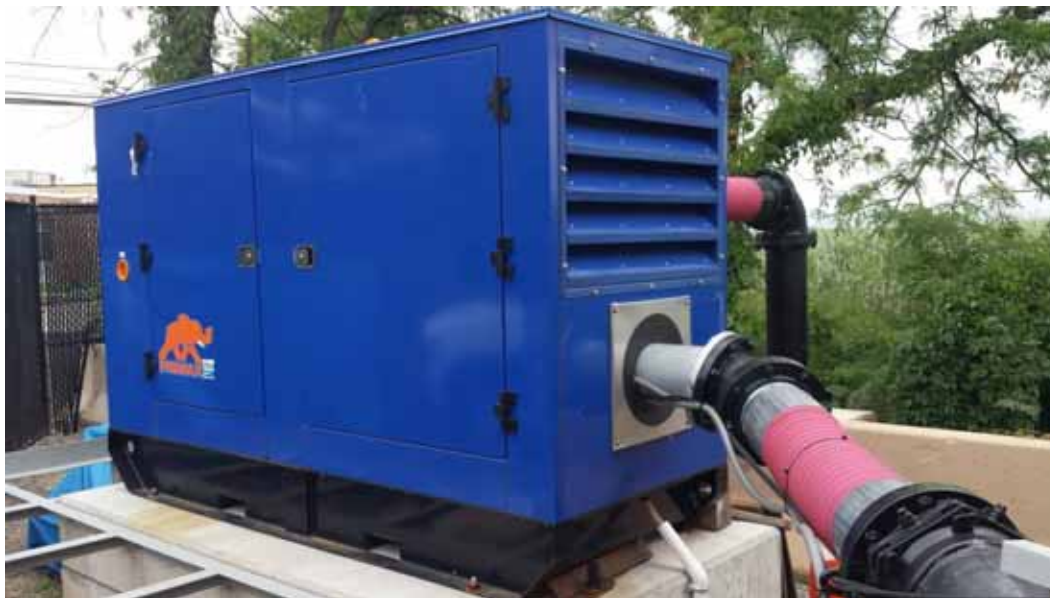
Figure 6: View of Primax backup pump
