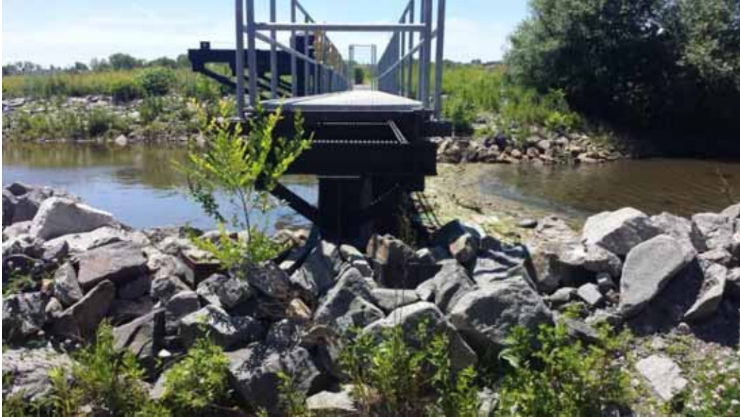
Figure 1: Side view of tide gate
