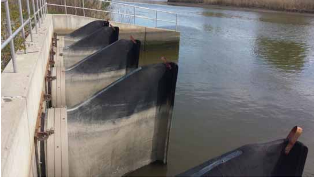
Figure 1: Downstream view of tide gate
