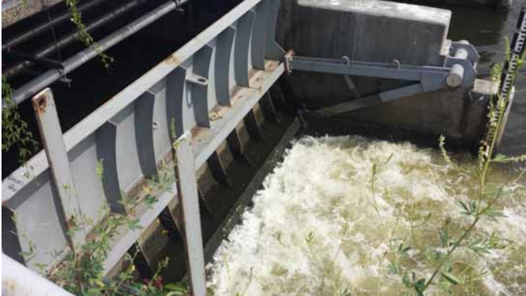
Figure 5: Close up of bascule gate
