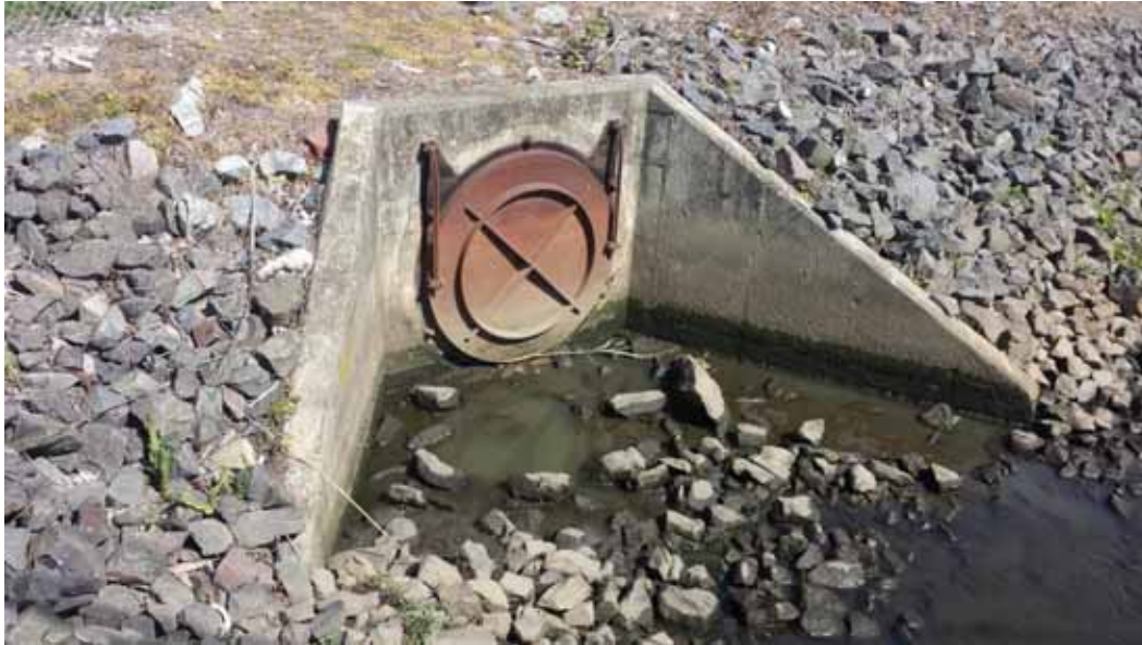
Figure 1: Upstream view of tide gate
