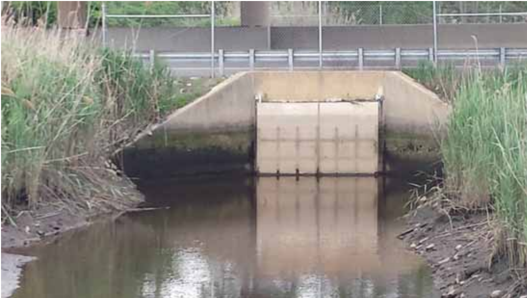
Figure 2: Upstream view of tide gate from bridge
