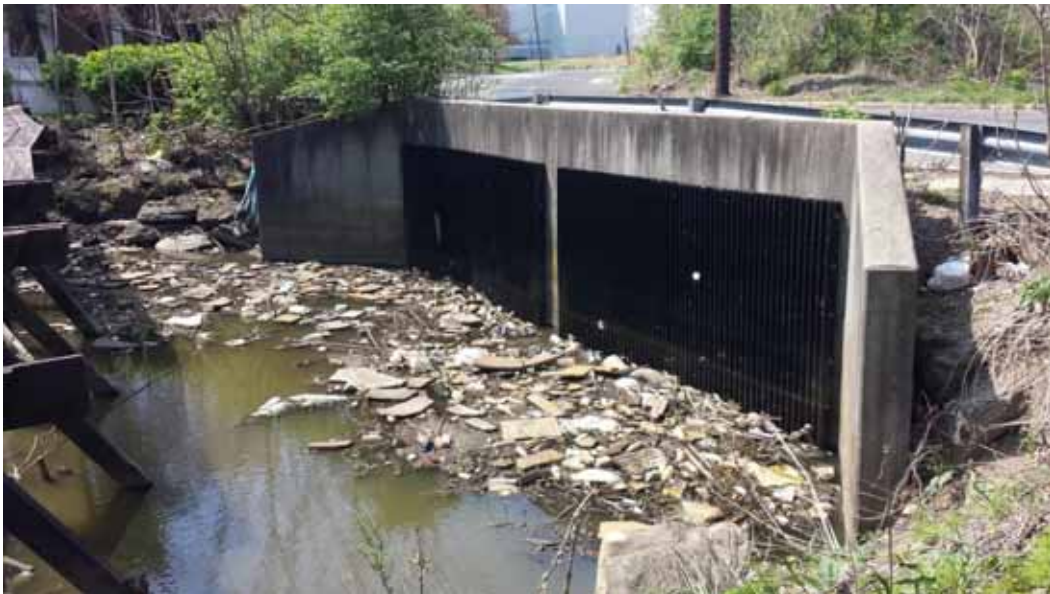
Figure 2: Downstream view of trash rack
