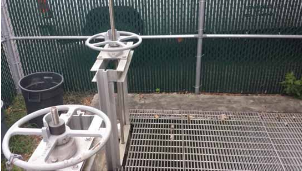
Figure 5: View of tide gate controls
