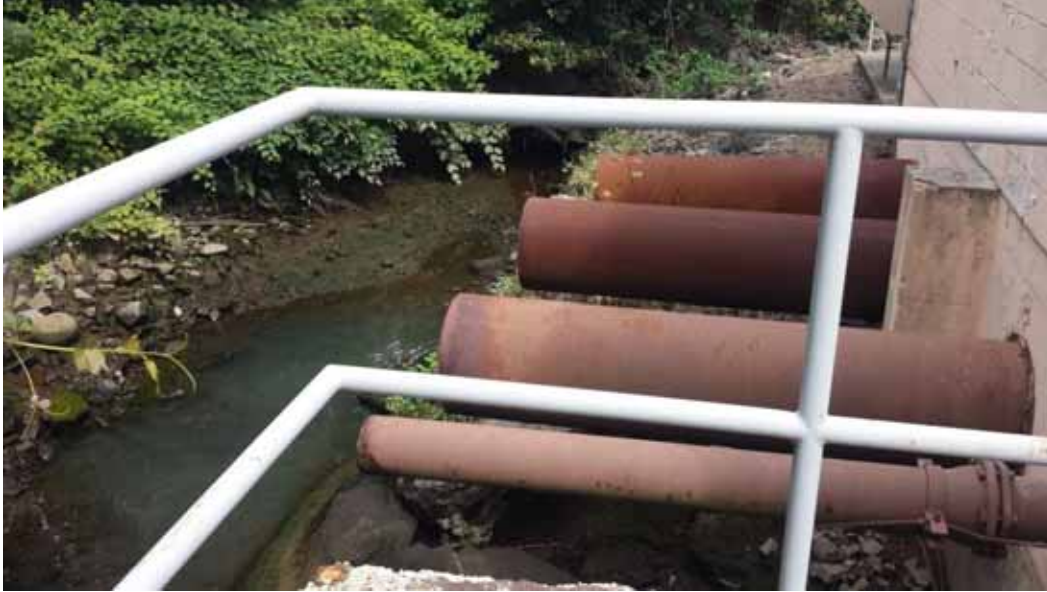
Figure 3: Pump outfalls
