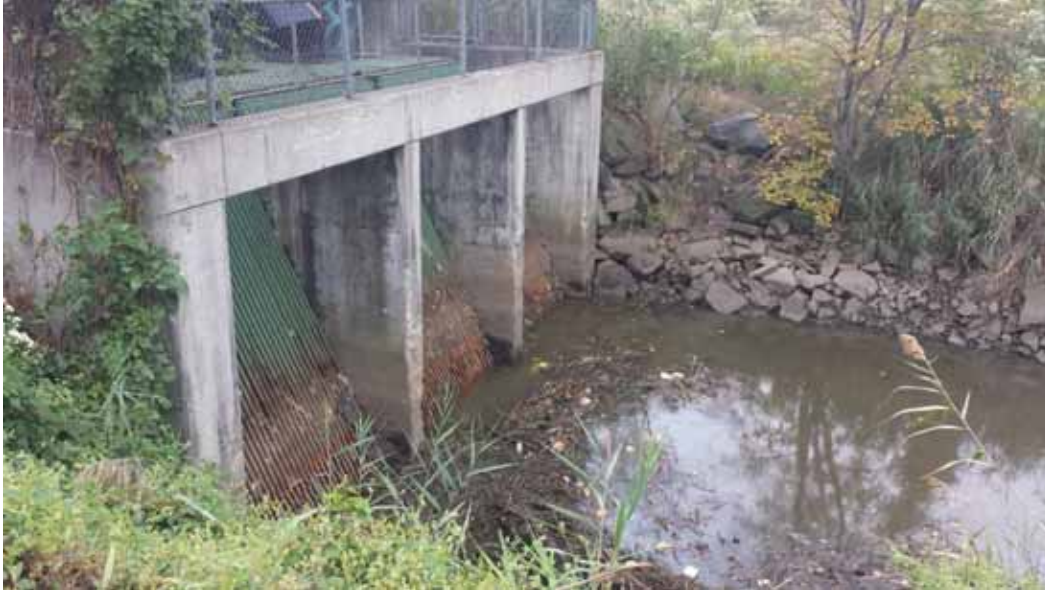
Figure 1: View of trash racks
