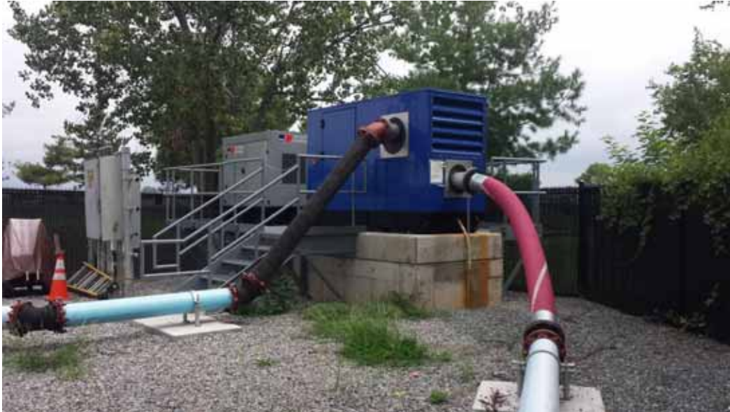
Figure 1: View of Primax above grade pump
