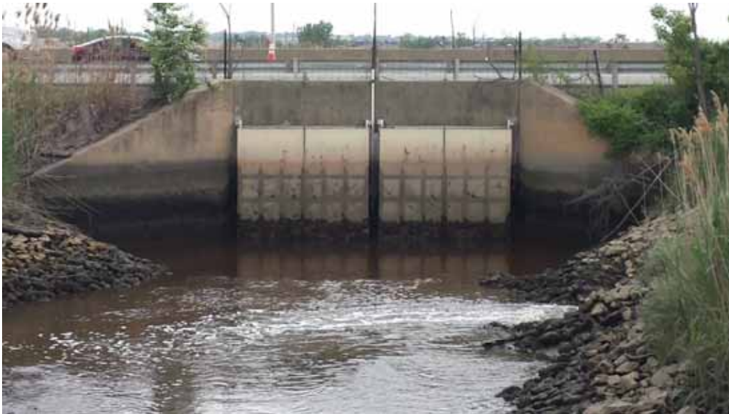
Figure 2: Upstream view of tide gate
