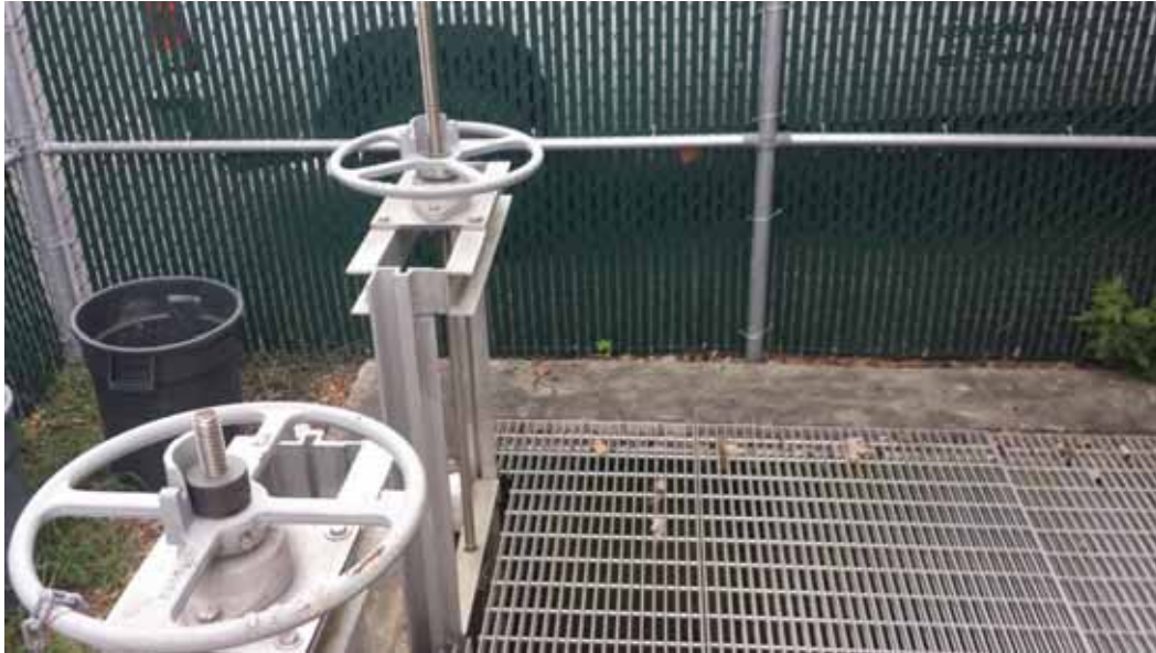
Figure 5: View of tide gate controls
