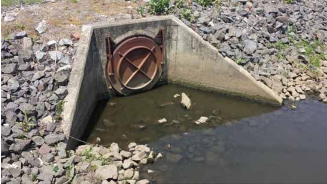
Figure 1: Upstream view of tide gate
