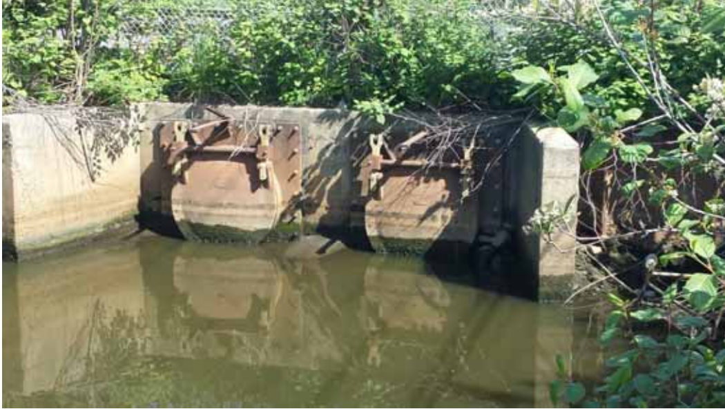
Figure 1: Upstream view of tide gate
