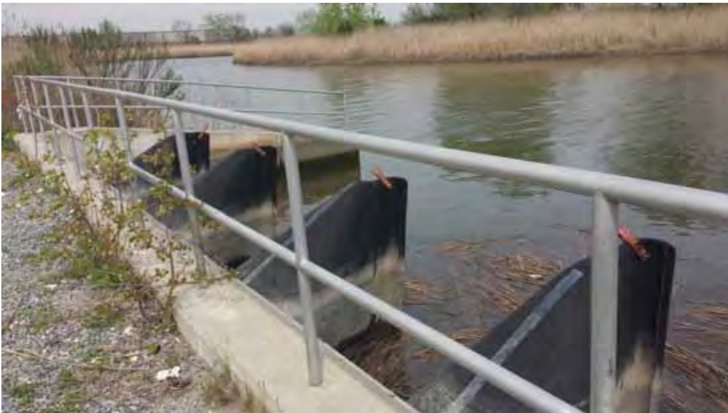
Figure 2: Downstream view of tide gate
