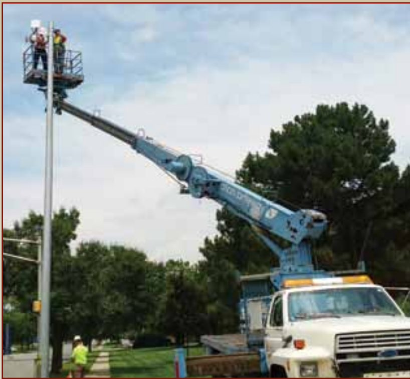
Installation of wireless communication transceiver
