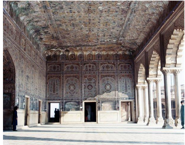
Fig. 5 Shish Mahal of the Shah Burj Complex, designed with openings for free circulation of air.
