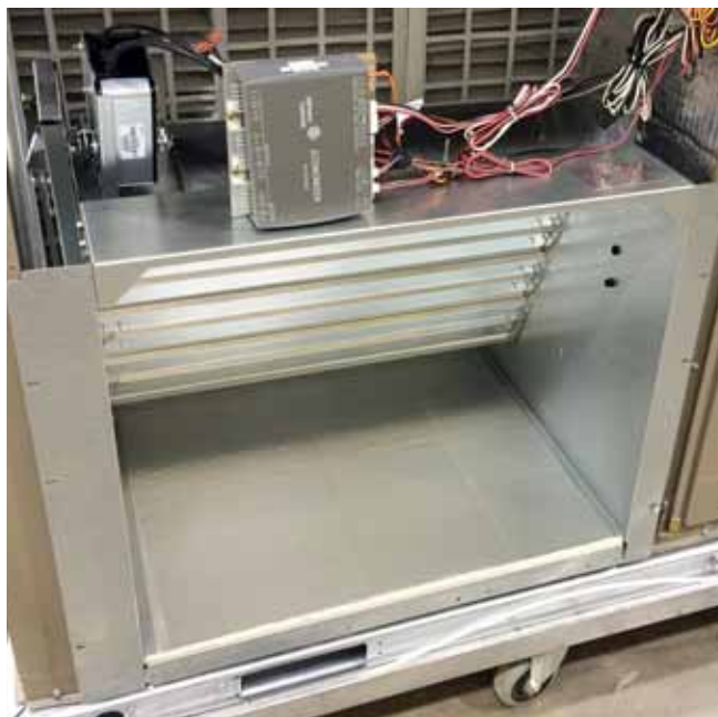
Figure 4 - Slide the fresh air damper into the unit
