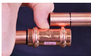
7b. Check the depth mark
