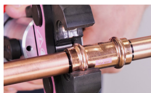
9. Align jaws squarely on the fitting
