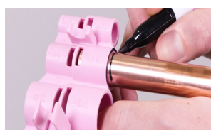
7a. Mark insertion depth on tube using depth gauge
