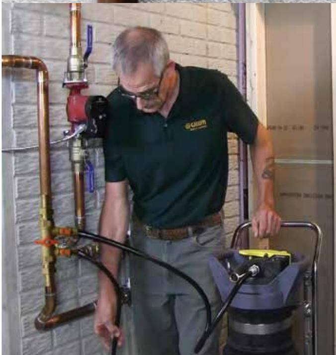
One is to install three ball valves, as shown in figure 4-4a. Another is to install a check valve in combination with two ball valves, as shown in figure 4-4b. The pressure differential created by the purging flow holds the check valve in its closed position.
