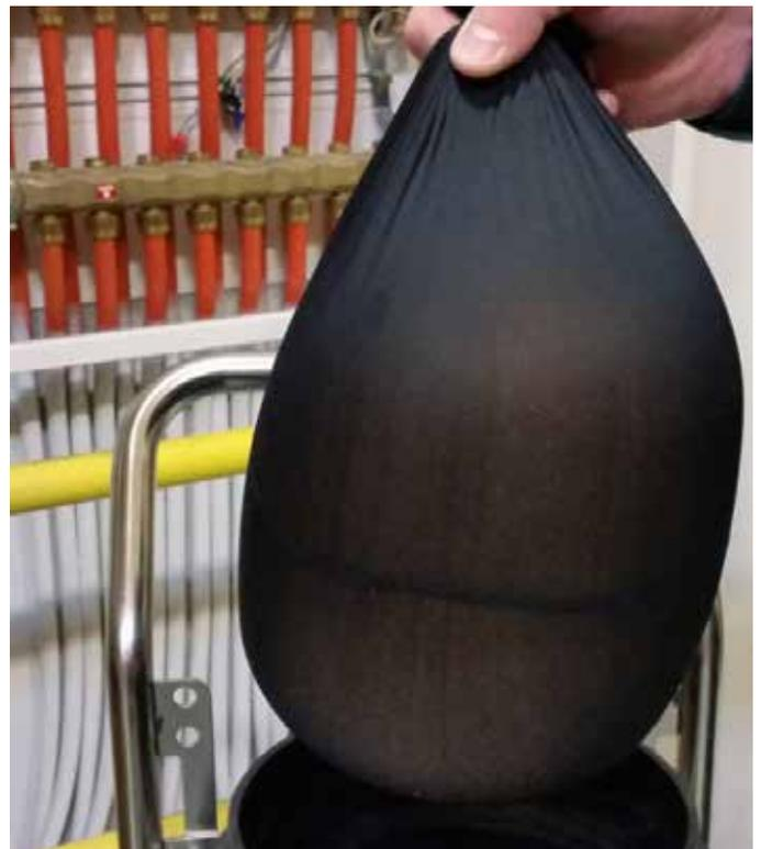
The smaller HYDROFILL holds two resin bags. The larger HydroFILL column holds 4 bags. Once the resin within these bags is “spent,” the head of the HYDROFILL is opened and the bags are lifted out. These bags only contain polymer resin beads and the ions that have been stripped from the site water. These are the same ions that were present in the site water. The spent resin bags can be disposed of in recyclable trash.
