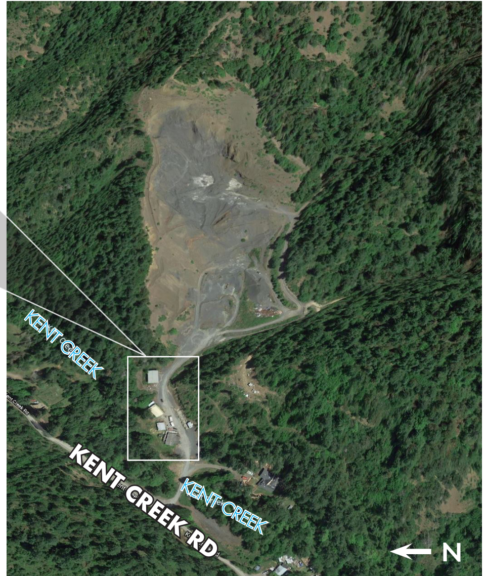
Aerial of Kent Creek Quarry looking East.
