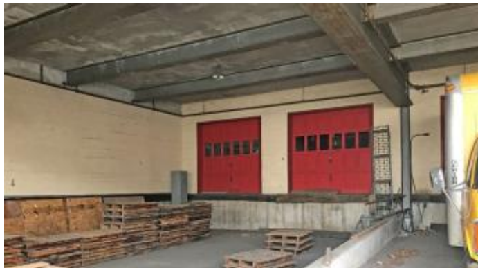
TWO INTERIOR DOCKS AT 4'
