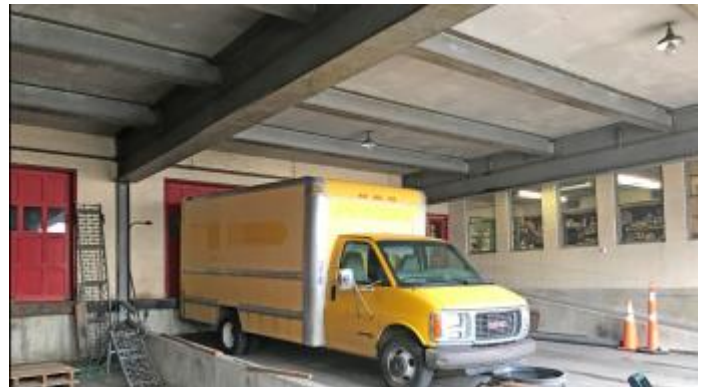
TWO INTERIOR DOCKS AT 3'
