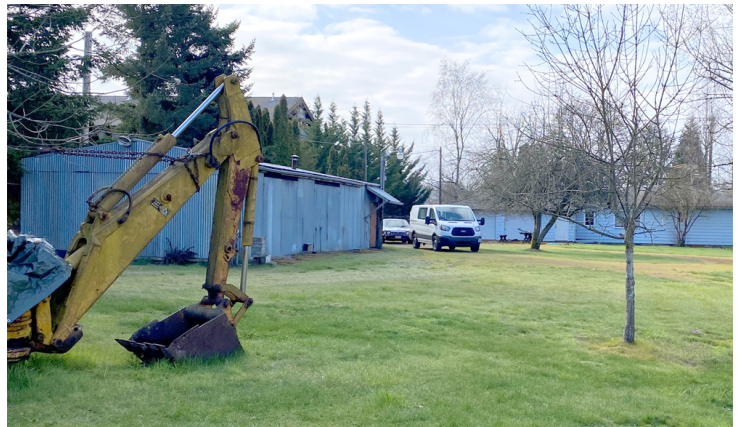
Small Pole Barn - Tear Down
