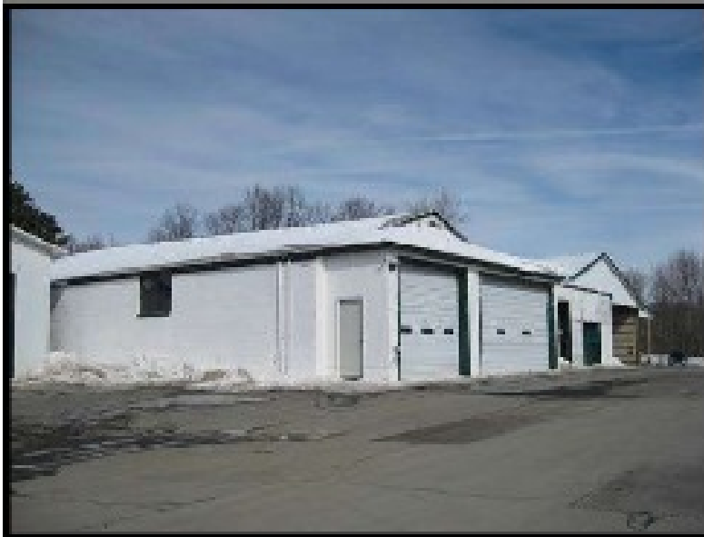
Bus Garage Building #2
