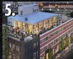
5. FOURTH & TRACTION (Offices/Retail/Restaurants) 32,000 SF of creative office space & 10,000 SF of Retail spaces.
