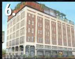
6. SOHO HOUSE (Hotel / Bar) A Members-Only club that will include 1,500 SF performance space, a 14,000 SF public market, a rooftop pool/observation deck and 36 guest rooms.
