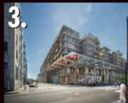
3. THE FORD FACTORY BUILDING 257,000 SF office building leased by Warner Music for the next 13 years. Will open fall of 2018.
