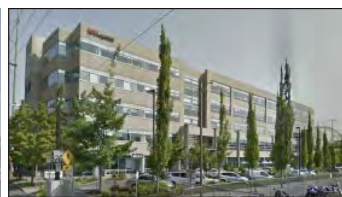
XPO OFFICE BUILDING
