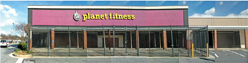
EXISTING PLANET FITNESS & SHOPS D SIDE (WEST) ELEVATION SCALE: NOT TO SCALE
