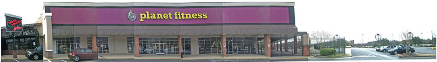
EXISTING PLANET FITNESS & SHOPS D FRONT (NORTH) ELEVATION SCALE: NOT TO SCALE
