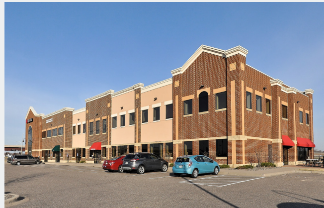
Back of Building
