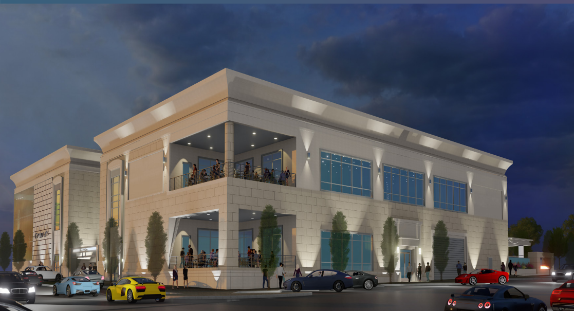
NORTH SIDE VIEW
