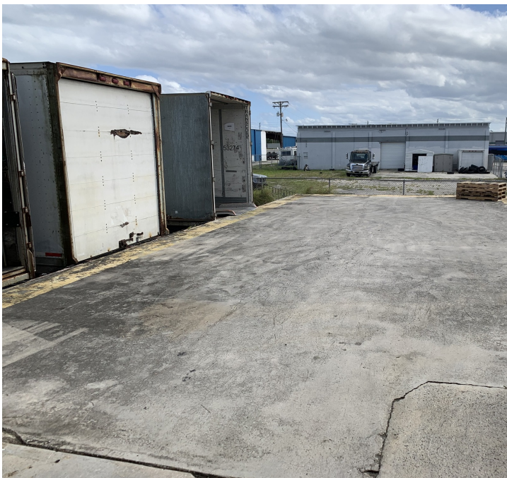
Loading Dock Platform (south side)
