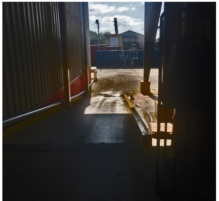
Transition Ramp (dock high to grade level)
