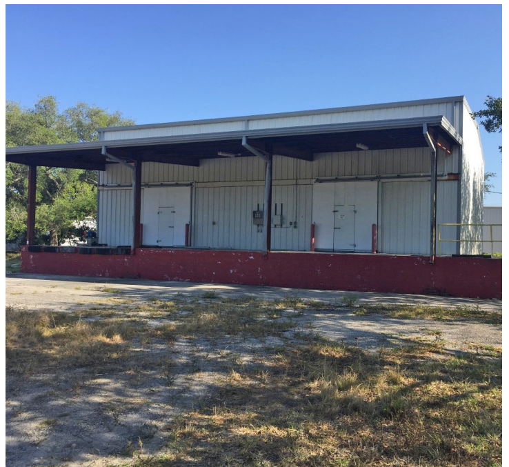
Stand Alone Cooler Building
