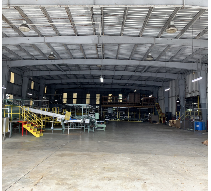
14,000 SF Structure (north end of complex)
