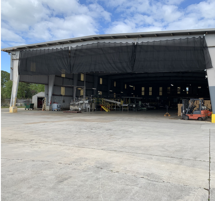
14,000 SF Structure (north end of complex)
