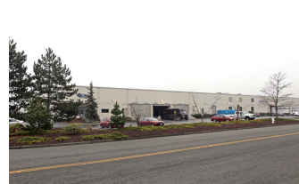
Matson/O'Neil Building 7043-7059 S 190 th St, Kent, WA 98032
