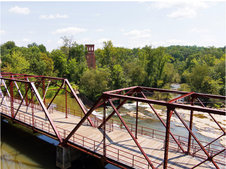
Glendale Shoals Bridge
