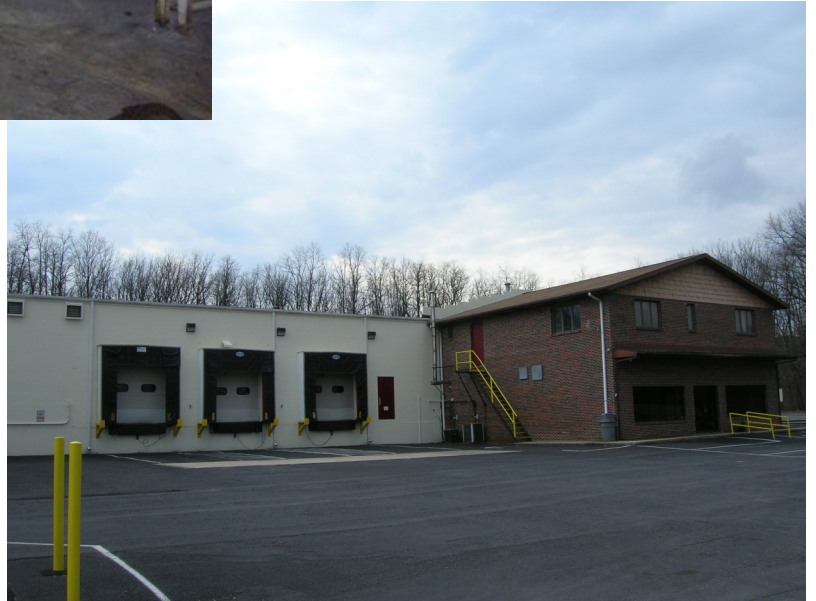
5 Docks (oversized) & 1 Drive-In Door
