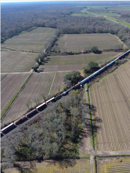
FACING WEST, VIEW OF UNION PACIFIC RAILWAY
