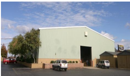
Rear Bldg. 1, 12,200 SF, Clear Span
