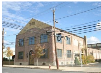
Two Story Office, 13,565 SF
