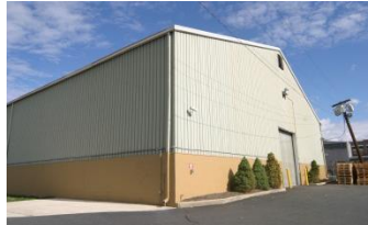
Rear Bldg. 3, 44,574 SF, Clear Span
