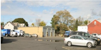
Repair Facility, Bldg. 4
