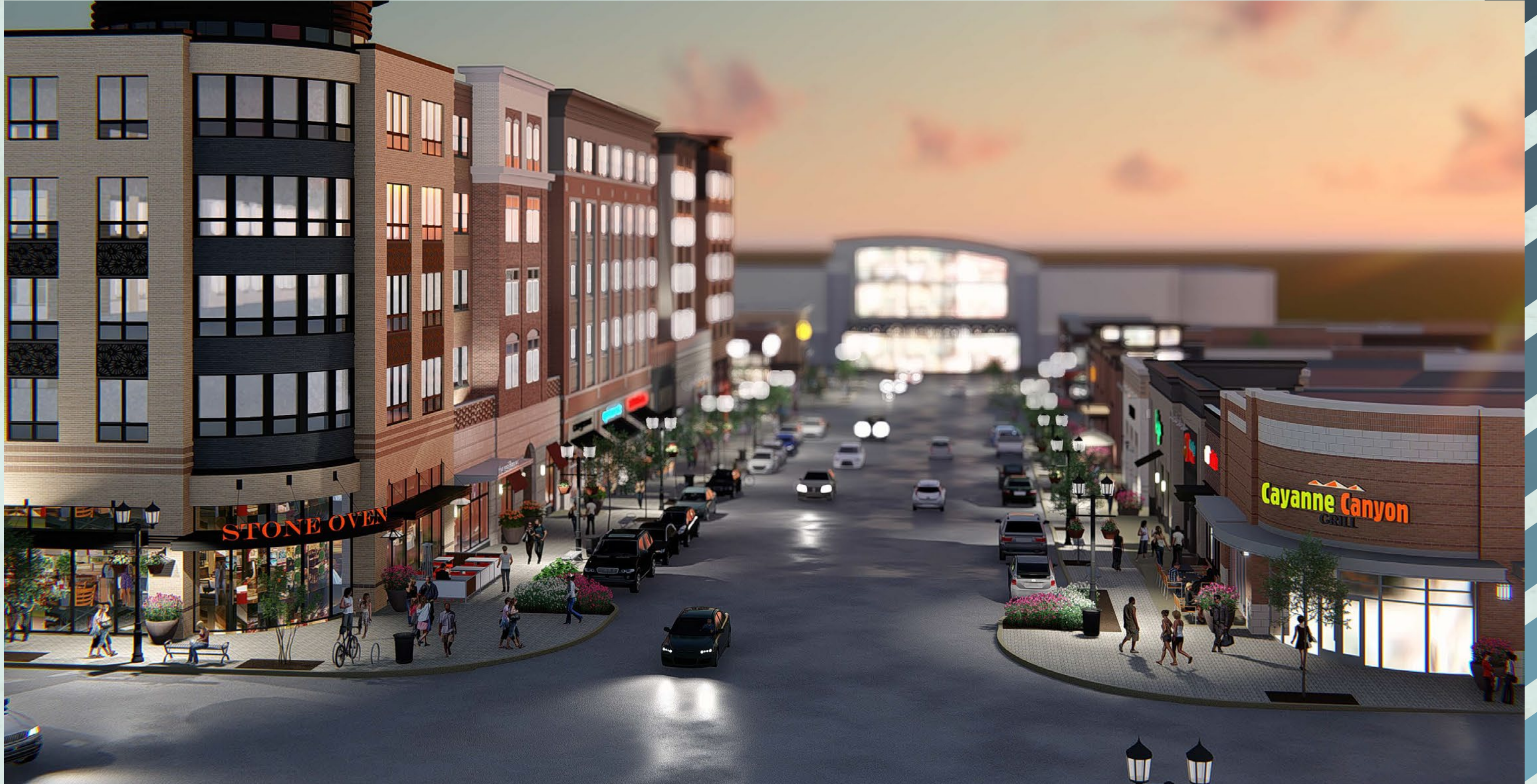
Looking south down Travis Lane (newly extended)
