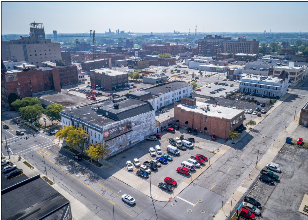
Southeast Elevation – Jefferson Street & 10 th Street
