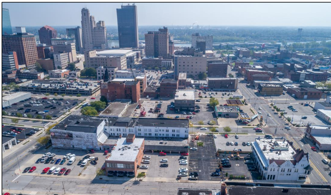
East Elevation – Central Business District view
