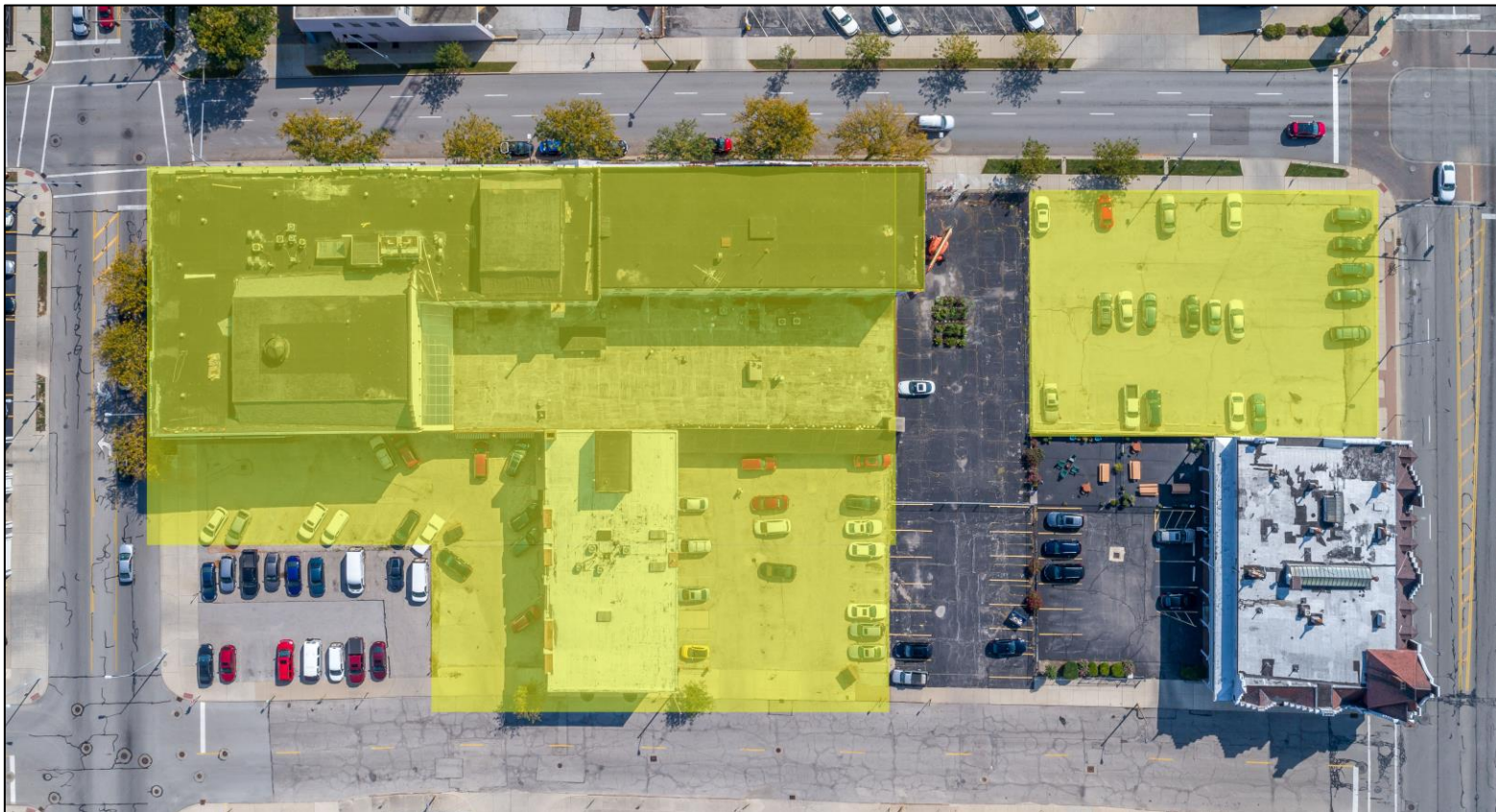
Overhead Aerial – Highlighted property view
