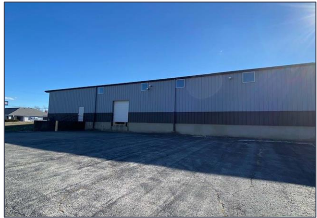
North elevation with truck dock
