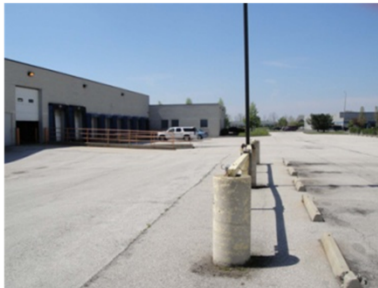
Block heater island
