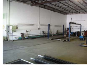
Mid section drive-in bay
