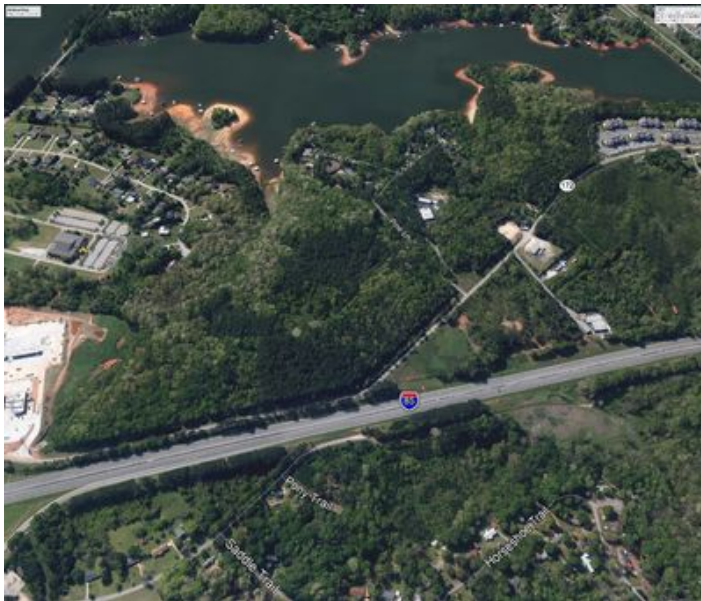
Aerial - From Interstate 85
