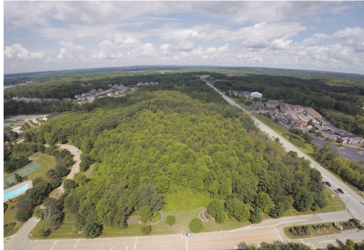
South end of property
