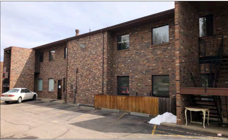
Back of Building
