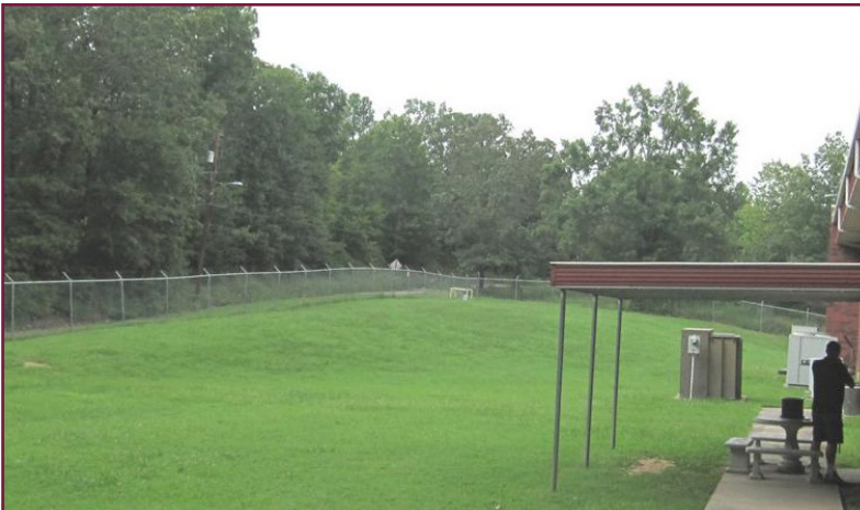
Building 2 - Office/Warehouse Fenced + Yard
