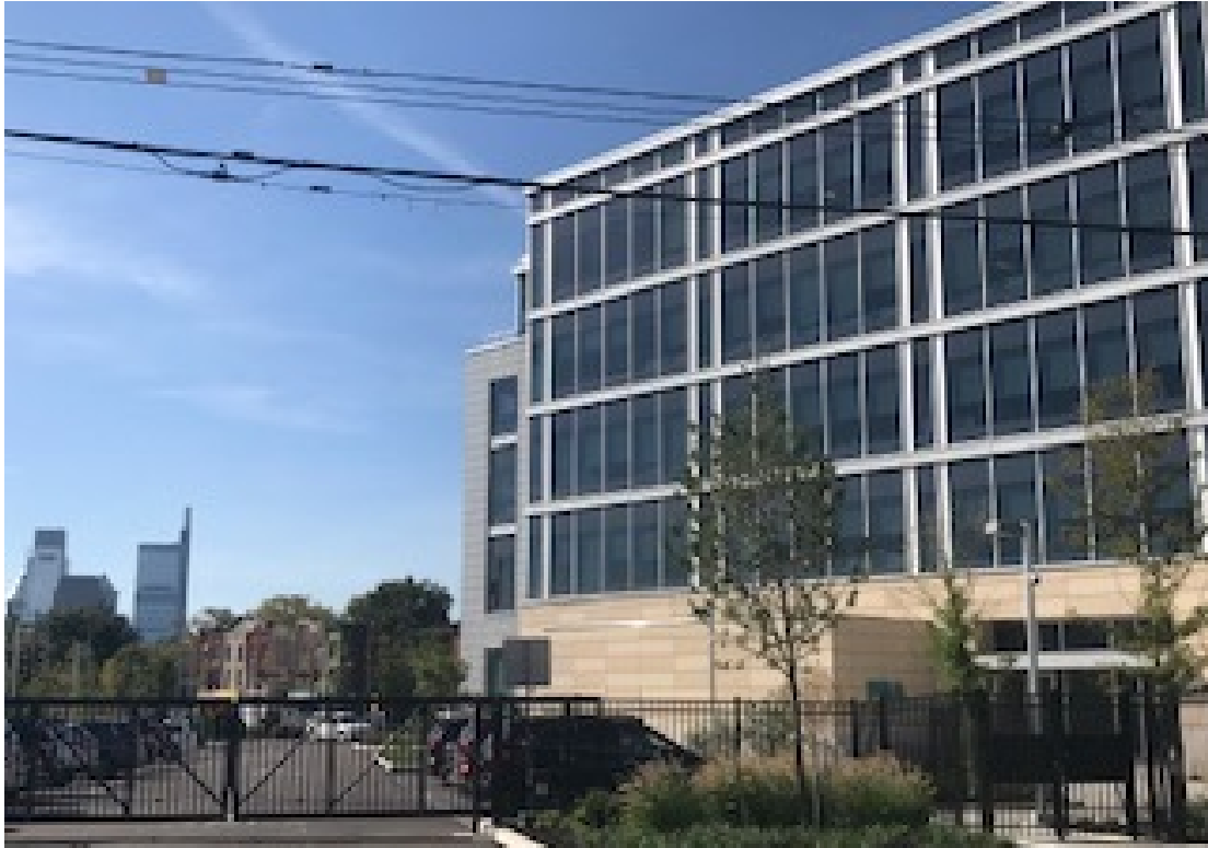
2013 Ridge Back of the Building
