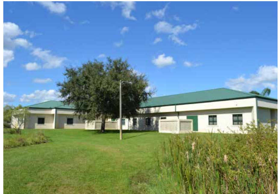
View of the building of the rear of the building facing northwest
