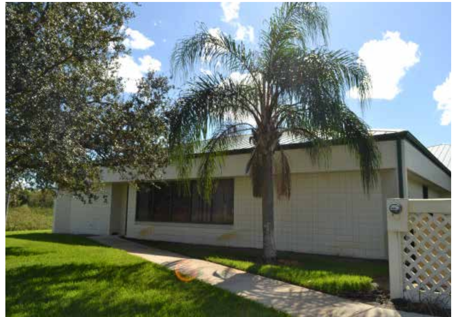
Shaded walkway along the northside of the building
