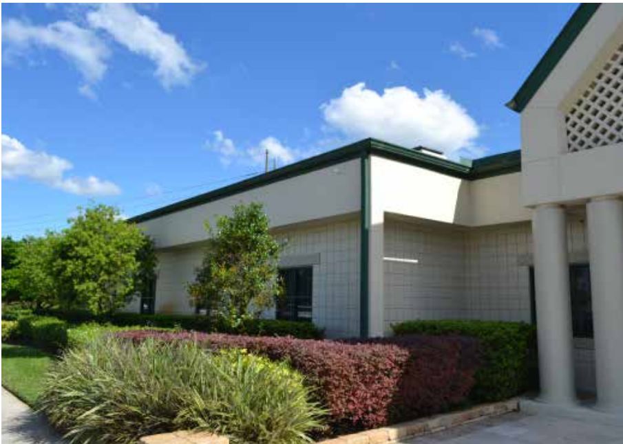
Beautifully manicured landscape at the front of the building
