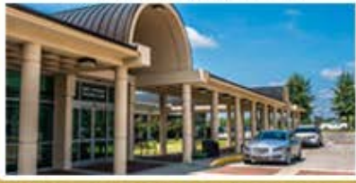
Southwest Georgia Regional Airport
