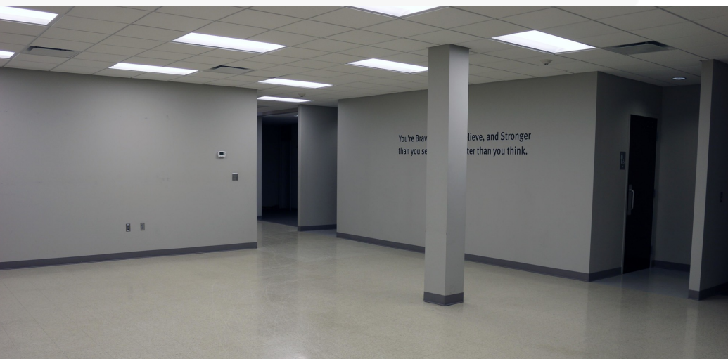
Space 324 - Open Space & Restrooms
