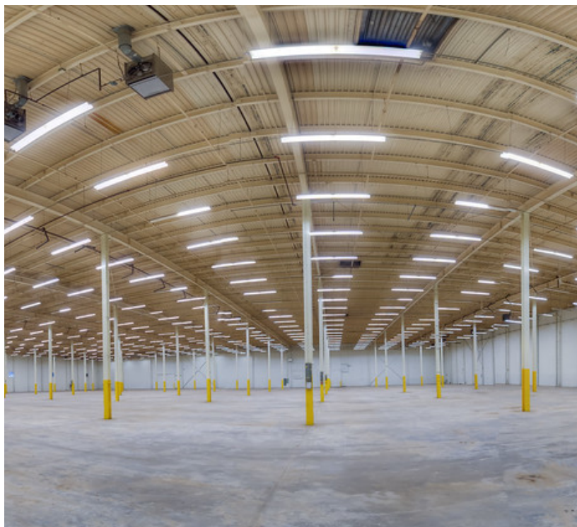
Phenix Center II, typical interior
