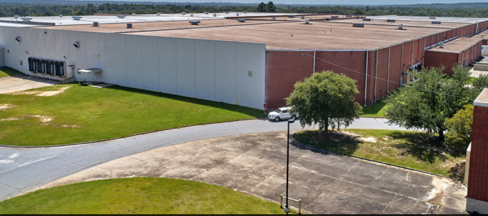
Phenix Center II north side
