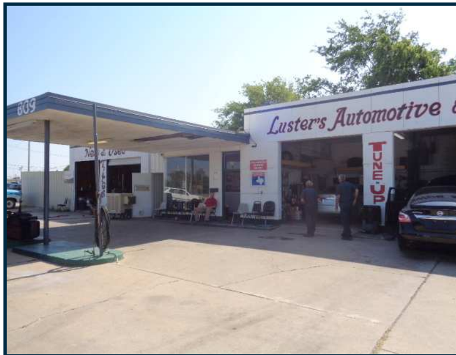
View of property looking north
