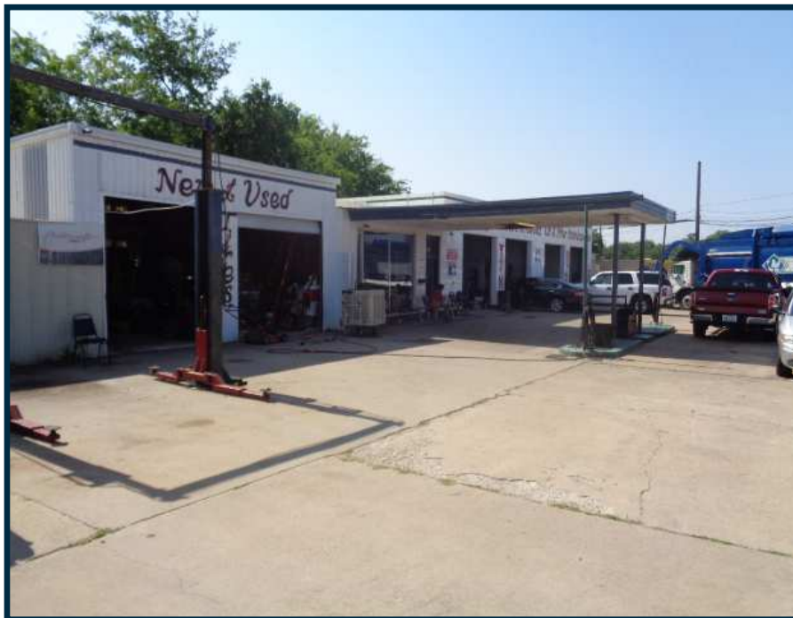
View of property looking south-outside lift stays
