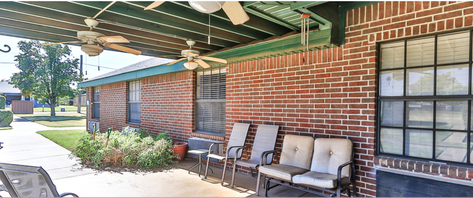
Back Porch Area
