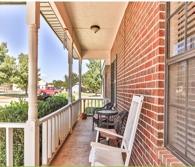
Front Porch of Independent Living Apartment
