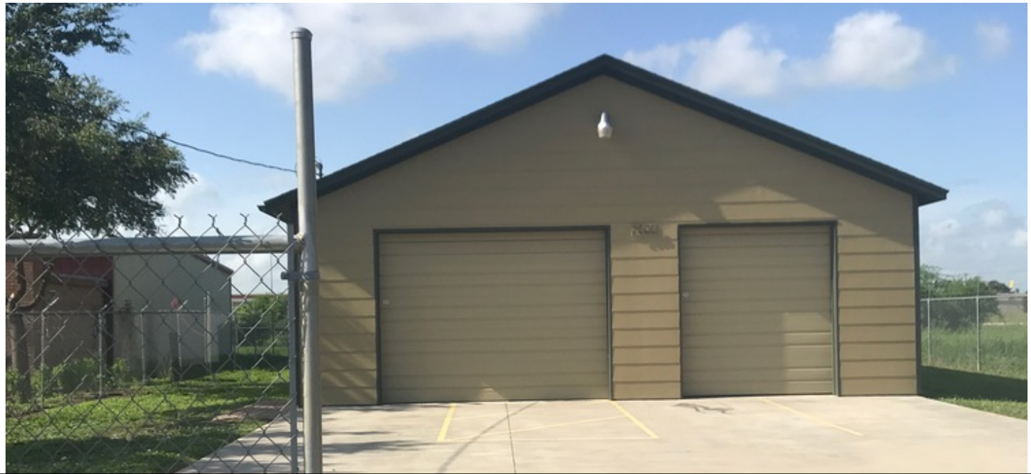
Front Facade with Barbed-Wire Fence
