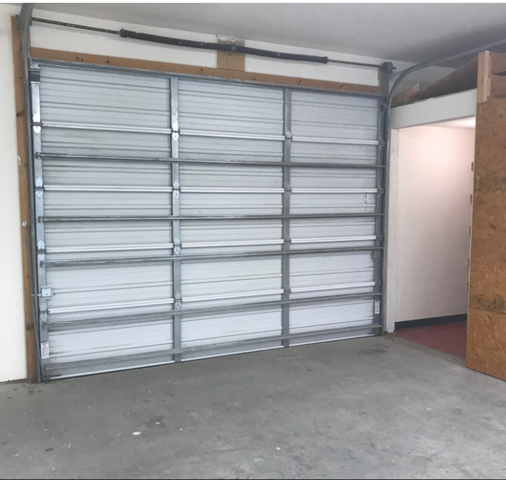
South Grade Level Door
