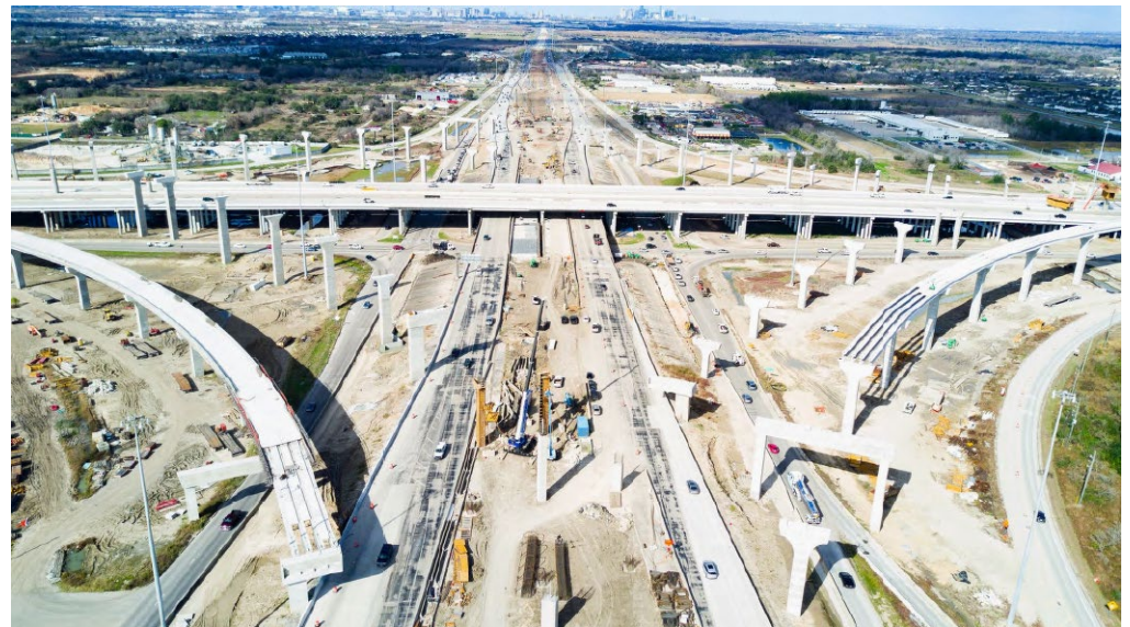
SH-288 at Beltway 8 Expansion Underway
