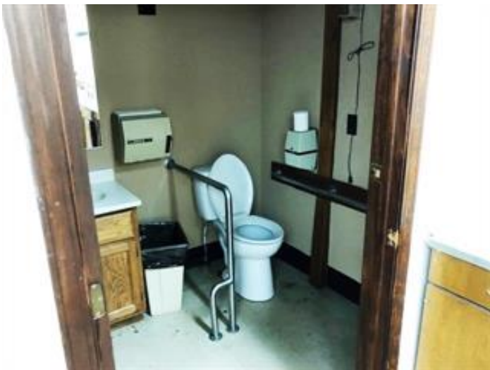
6th street showroom inside ADA RR
