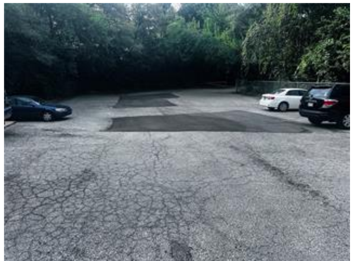
rear outside storage area
