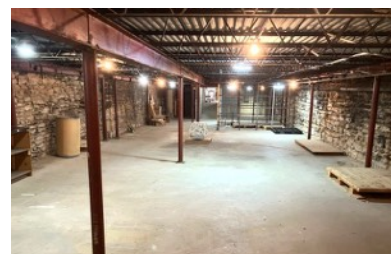
Basement View to Building Rear
