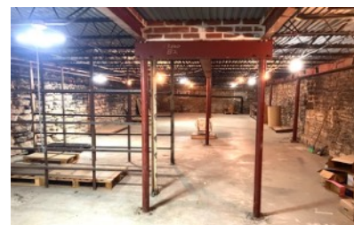
Basement View to Building Front
