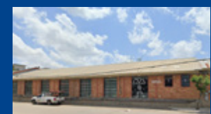
Office building 2220 Commerce St
