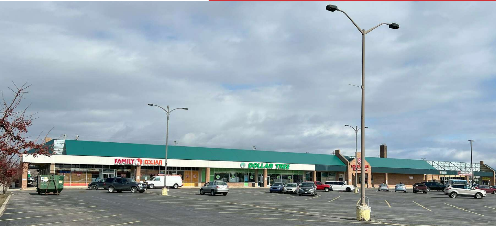
North Side of Strip Center
